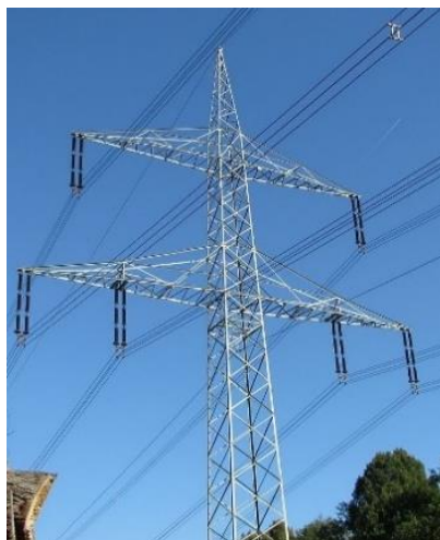
Figure 2.1: Danube tower for a transmission line of 380 kV
